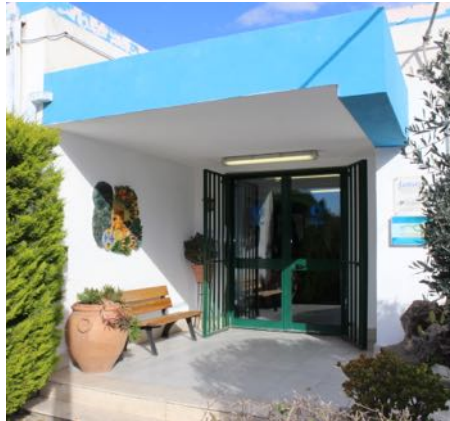
Fig. 12: Entrance of the ACE Headquarter.
